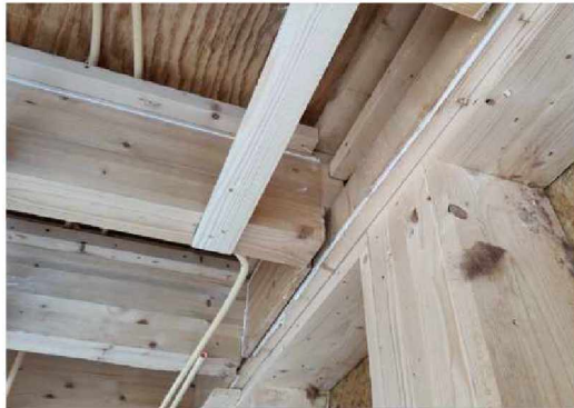
Oplegging houten balklaag
