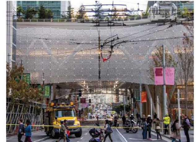
Transbay Transit Center, San Francisco
