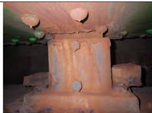
Detailfoto 13: Oplegging 3 links
