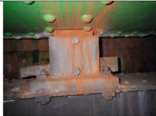
Detailfoto 9: Oplegging1 links
