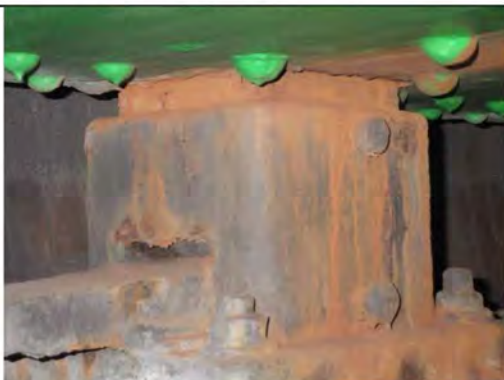
Detailfoto 12: Oplegging 2 links
