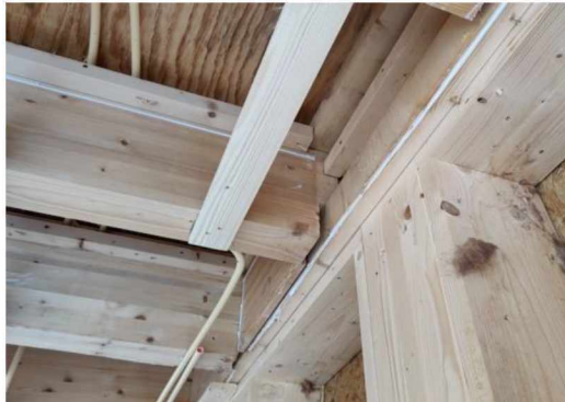
Oplegging houten balklaag
